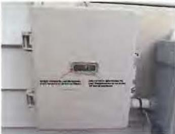
fifteen minutes. During this period, a red light appears on the control unit. After the fifteen minute period the air conditioner returns to service and a yellow light appears on the control unit. This process
