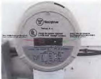
Participants have a load control unit installed on central air conditioning units. When the electric demand is high the City will cycle the air conditioner and in exchange participants receive a four dollar credit on electric bills during the months of May-September.
