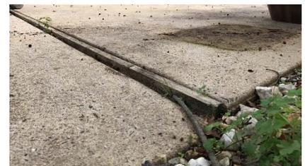
sidewalks may pose a tripping hazard or be out of compliance with ADA regulations. When that's the case, property owners will be required to make repairs, or in some cases, replace the damaged portion of the sidewalk.
